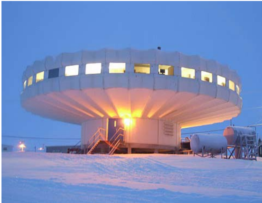
Plate 8 "The Lab," or Eastern Arctic Research Center, Igloolik, constructed in 1975. The effort to involve the community in Arctic science included a competition to give the laboratory a local name. The winning entry recognized the building's resemblance to a Snowy Owl , 1988. Photo: Michael Bravo
